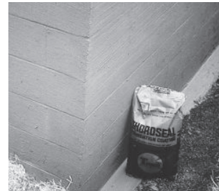
Sealed and waterproofed.
